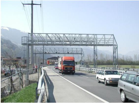
Furthermore, the FOCBS checks that the HVC declaration is correct with fixed and mobile monitoring points in traffic. The data from the recording devices is transmitted via the DSRC radio link by the current 27 fixed monitoring installations on the Swiss motorway network and is automatically compared with the data (number plate, vehicle length, etc.) captured electronically by the installation.
